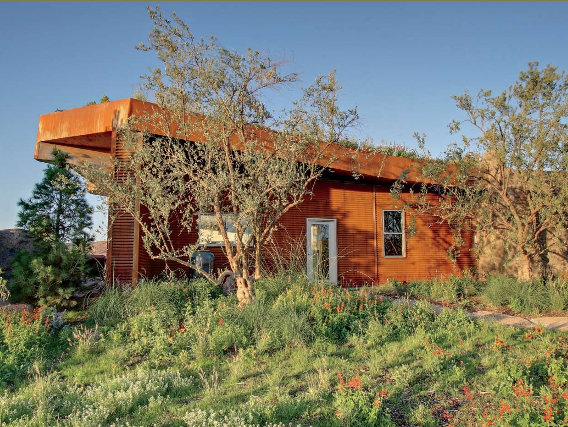
Carlson planted the prairie-style roof of his meditative desert getaway to look as though the house had just risen from the ground. The chemically-rusted corrugated steel skin both insulates the house and blends with the boulders.
